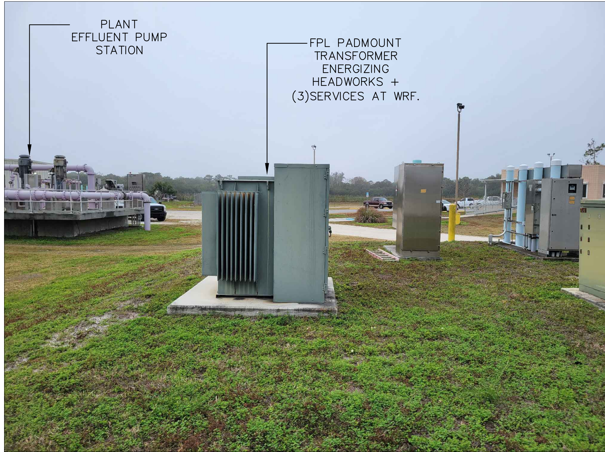
EXISTING 480V, 3P FPL ELECTRICAL SERVICE TRANSFORMER TO REMAIN N.T.S.
